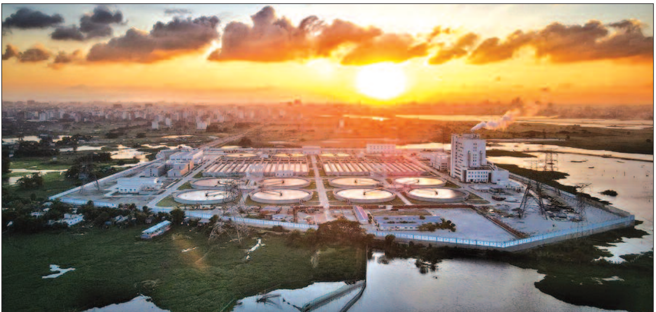
Aerial photo taken on Aug. 24, 2022, shows the China-funded Dasherbandi Sewerage Treatment Plant in Dhaka, Bangladesh. (Xinhua)
